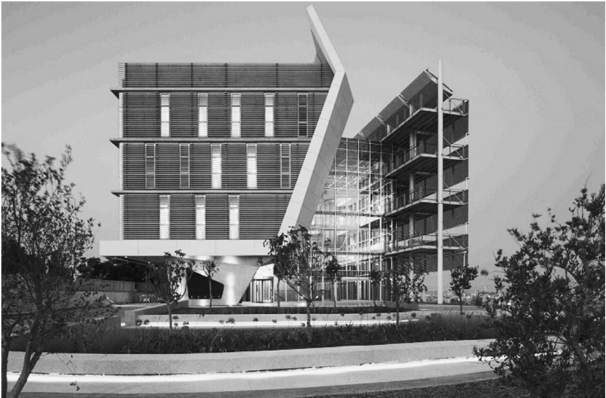
Figure 2.6 The Porter School of Environmental Studies is Israel’s First LEED Platinum Building. It is conveniently located within walking distance of public transportation – Tel Aviv University Railway Station and a bus terminal. The building’s sustainable features include solar PV panels, wastewater recycling, a green roof, and an “EcoWall” with solar tubes that will provide heat during the winter while during the summer the same wall will provide shading to keep the interior cool.
