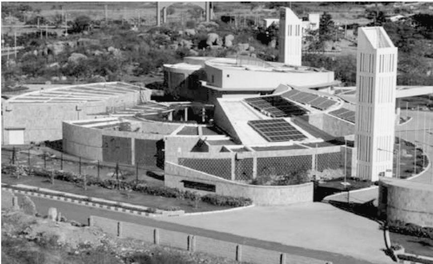
Figure 2.5 The Sohrabji Godrej Green Business Centre in Hyderabad, India. In 2001, this building encouraged the development of green building in the country. This was the first platinum-rated green building under the LEED rating system, outside the USA, boasting energy savings of 63%. Source: Confederation of Indian Industry.
