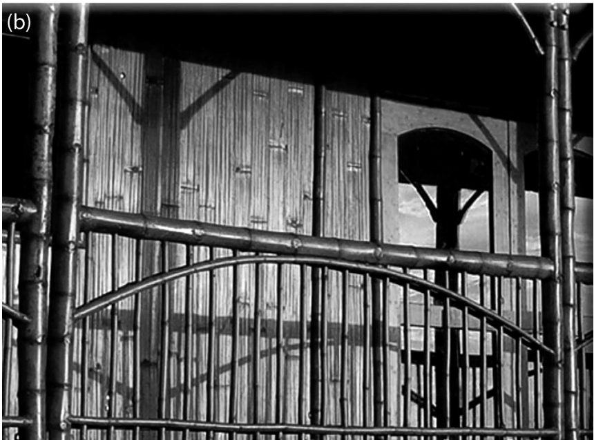
Figure 6.12 (a) Kitchen cabinets made from bamboo. (b) Photo showing use of bamboo as exterior siding. Source: Bamboo Technologies.
