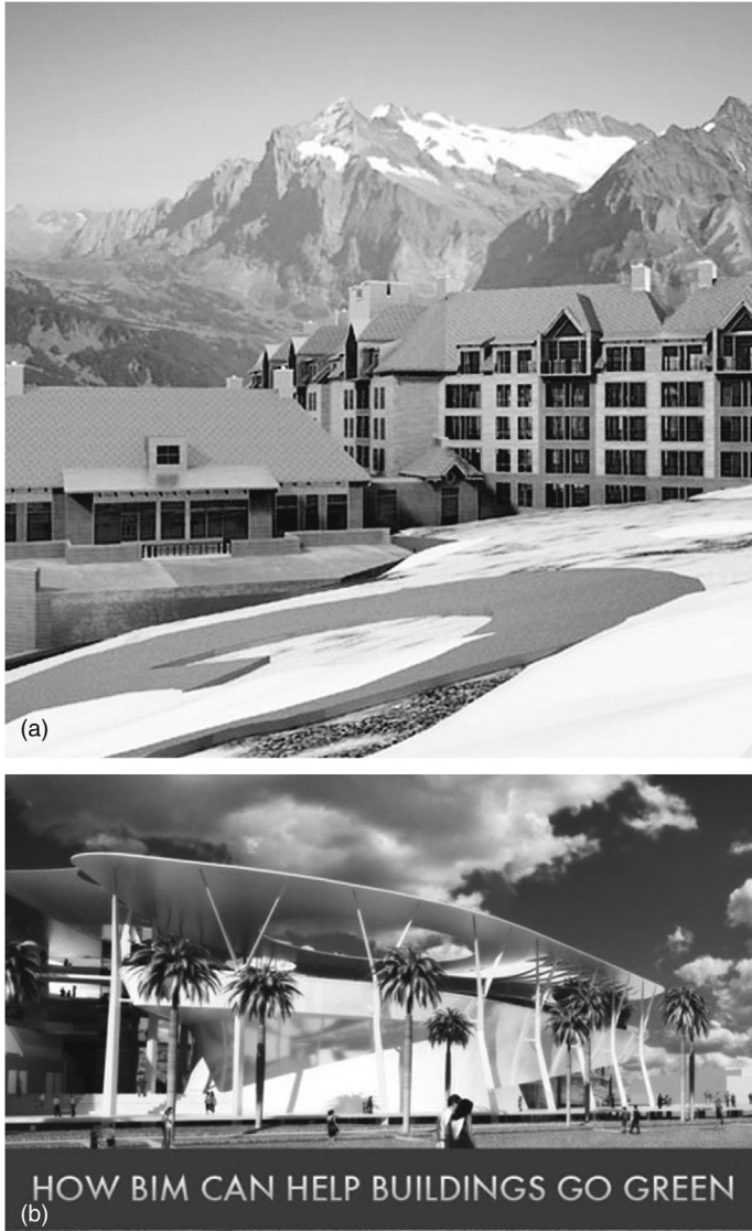
Figure 5.1 (a) Highlands Lodge Resort and Spa project, a joint venture of Q&D Construction and Swinerton Builders, Inc. where Vico, a BIM software package was used. The five-star hotel and high-end luxury condominiums have a total gross floor area of 406,500 ft. 2 (37,720 ft. 2 ) and are built on a roughly 20-acre site at the Northstar-at-Tahoe Ski Resort in Northern California. (b) Miami Science Museum, designed by Grimshaw Architects uses Building Information Modeling (BIM). The Miami Science Museum carefully integrates the direction and location of the sun into its design – engaging in both passive and active solar design strategies. Source: Part a, Vico Software Inc. Part b, Jill Fehrenbacher.
