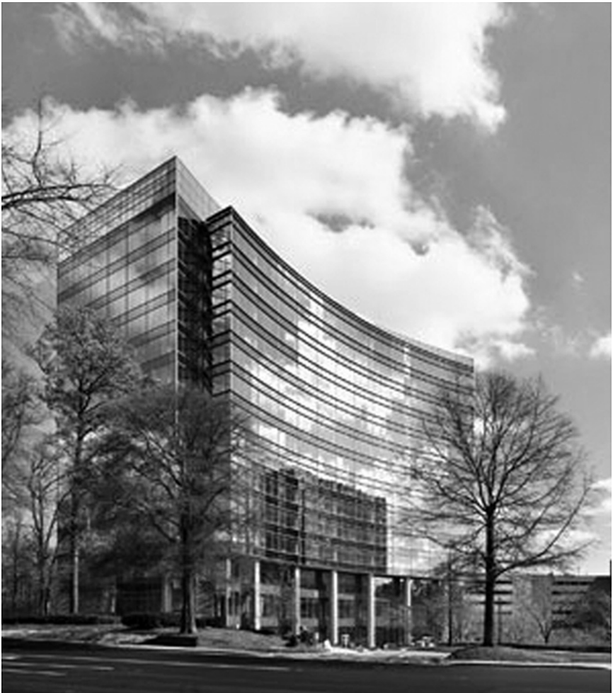
Figure 2.7 New 356,000-ft. 2 Newell Rubbermaid Corporate Headquarters in Atlanta, GA. This building achieved a two-globe rating using the Green Globes New Construction module. Courtesy: Green Building Initiative.
