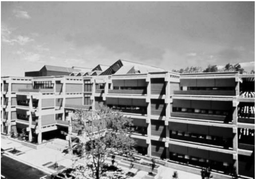
Figure 1.1 Photo of the Gregory Bateson Building in Sacramento, California (1978), which was a model energy-efficient state office building designed by Sim Van der Ryn and which employed several energy-saving tools, including an automated solar-tracking shading system with exterior ElectroShades®. Source: MechoShade Systems, Inc.
