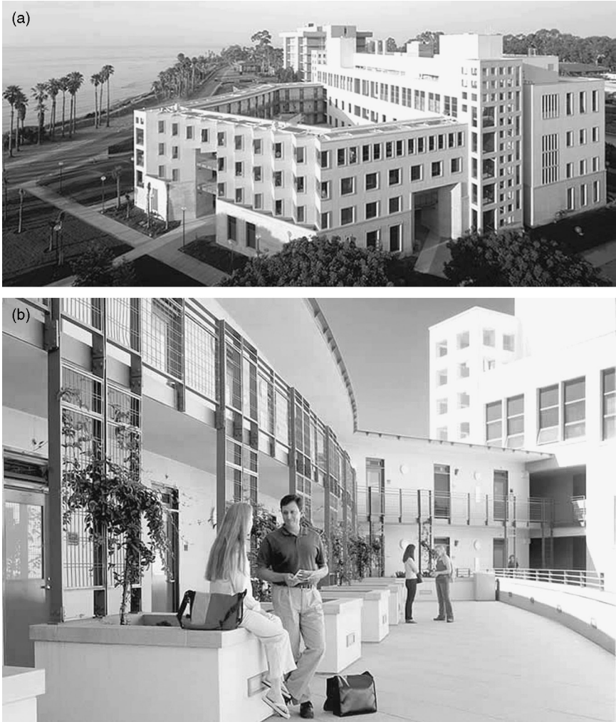
Figure 2.3 (a) Bird's eye-view of Donald Bren School of Environmental Science & Management at UCSB, which is a LEED Gold Pilot project. It utilized silt fencing, straw bale catch basins, and scheduled grading activities in accordance with the project's erosion control plan. (b) Bren Hall – faculty and students on the third-floor terrace. Source: Bren School website: http://www.esm.ucsb.edu/
