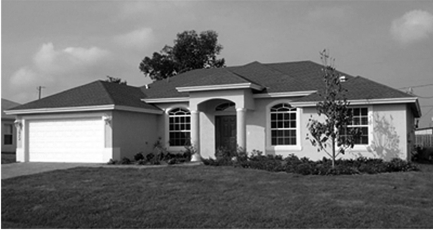
Figure 4.3 Photo of a Port St. Lucie (Florida) home that became the first in the state to earn a certification through the USGBC's LEED for Homes pilot program after several inspections and performance tests were completed by Florida Solar Energy Center. The home completed the certification process on March 19, 2007. Courtesy: Florida Solar Energy Center.
