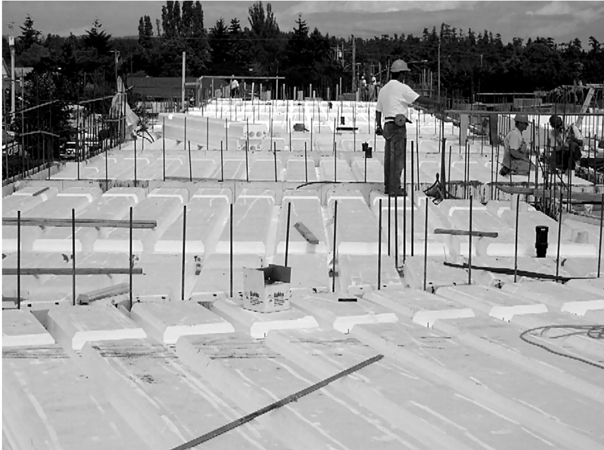
Figure 6.8 Photo Depicting Application of Insulating Concrete Formwork Quadlock System. Source: Quad-Lock Building Systems Ltd.
