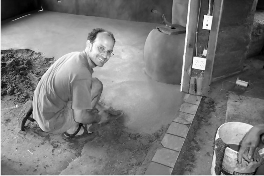
Figure 6.3 Illustration Showing Method for Installing an Earth Floor. Source: Dancing Rabbit.
