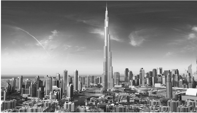
Figure 1.7 Illustration of Burj Khalifa. Known as Burj Dubai before its inauguration, it is the tallest man-made structure in the world, and stands at 829.8 m (2722 ft.). The building, which was designed by Skidmore, Owings & Merrill and developed by Emaar Properties, officially opened on January 4, 2010. The Symbol of Dubai skyscraper has more than 160 habitable floors, 57 elevators, apartments, shops, swimming pools, spas, corporate suites, Italian fashion designer Giorgio Armani's first hotel, and an observation platform on the 124th floor. The total estimated cost for the project is estimated to be about US$1.5 billion. Source: Skidmore, Owings & Merrill.
