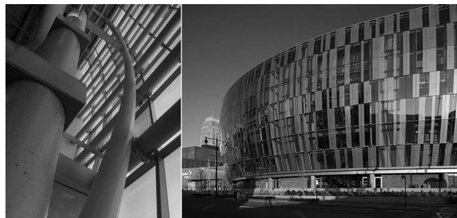
Figure 5. Fritted glass with vertical panels of clear glazing. Photo by Michael Spillers. The glazing between the fritted panels is acceptable vision glazing.
