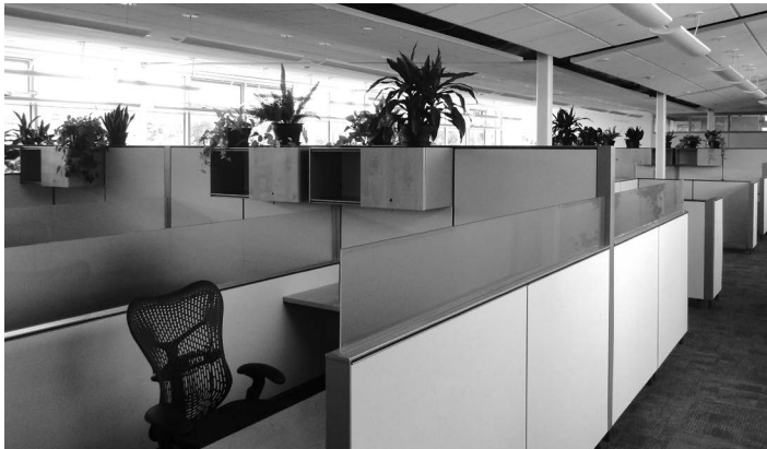
Figure 8. Partial-height partitions with frosted glass. Photo by Marcus Sheffer. Frosted glass is not acceptable because it interferes with occupants' views to the vision glazing.
